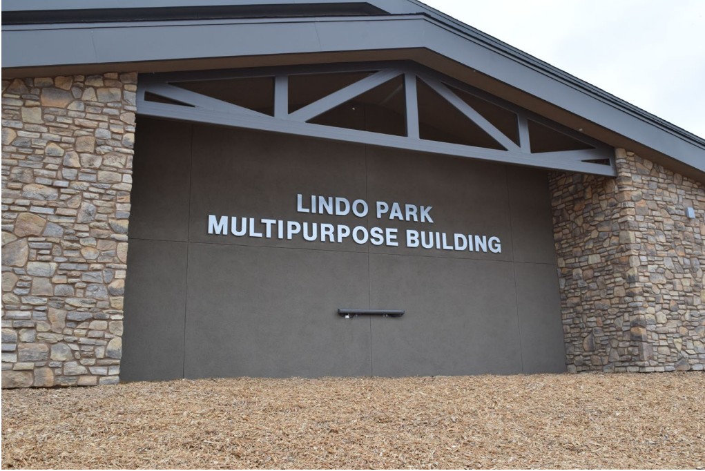
Lindo Park – Multipurpose Room and Kitchen Modernization
